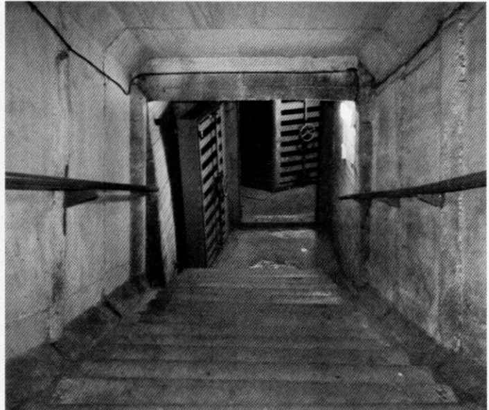
Airlock at the entrance to the ‘Shooting Bunker’
